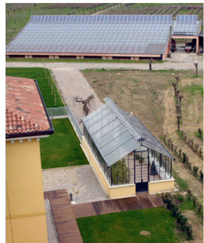
The Istituto Bacologico's solar station uses three photovoltaic modules in monocrystalline, polycrystalline and amorphous silicon of 20 kW each. To comply with the plant's requirements, Carlo Gavazzi provided custom-designed energy counters, power analysers and the interface protection, all of them devices that control the minimum and maximum voltage as well as the frequency.
