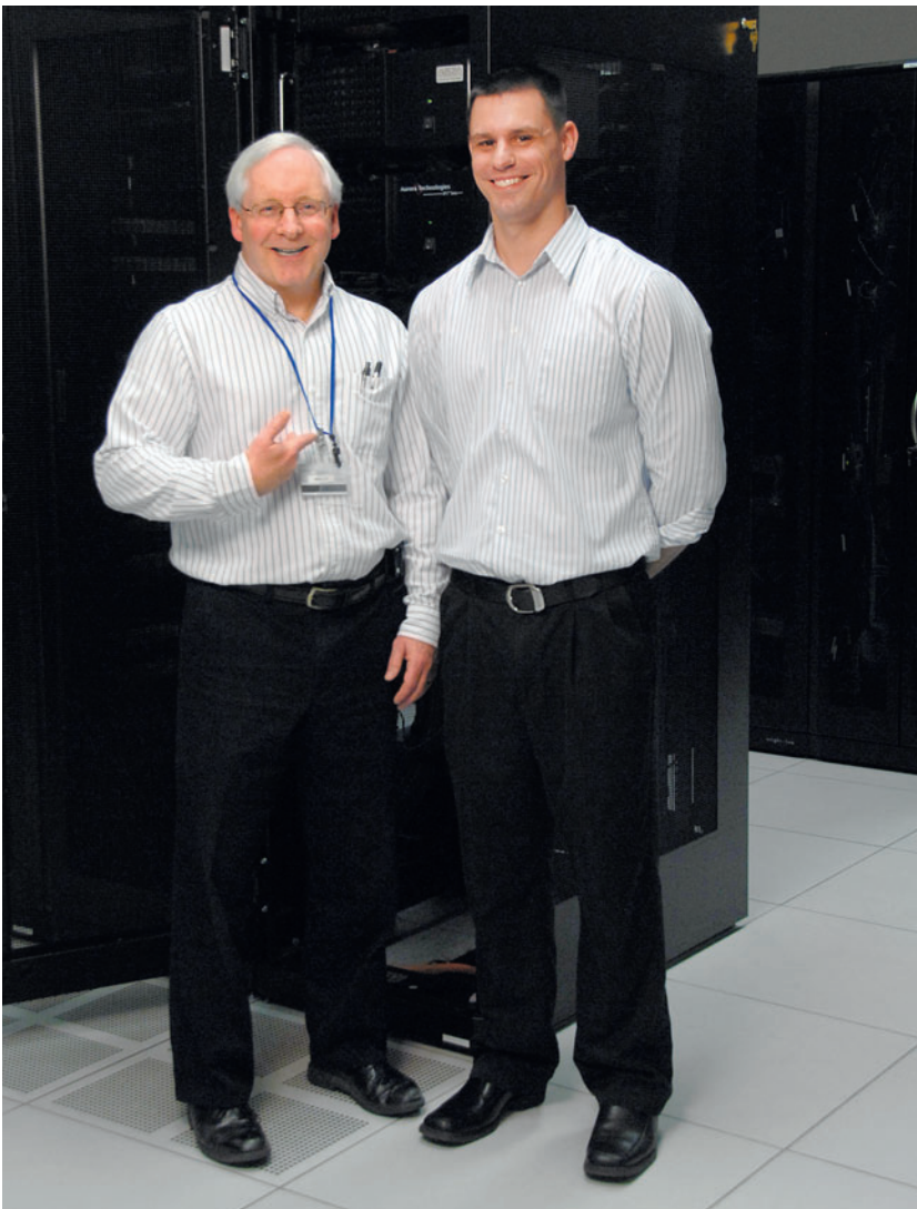
Sherman Layton of State Street and Greg DeCristofaro, Carlo Gavazzi's area manager discuss future requirements in front of cabinets containing Control Tower and PCI expansion chassis.
